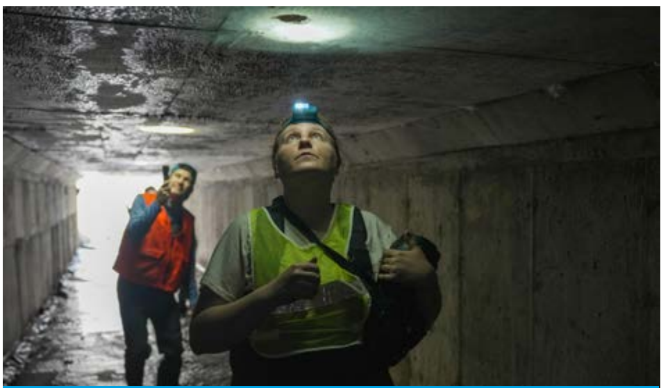
Molly Simonis searches for bats in a culvert under Interstate 85 in Lee County, Alabama.
